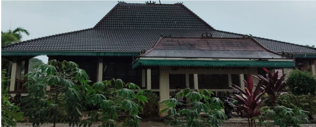
Figure 1. Banyuasin Regency Traditional House
